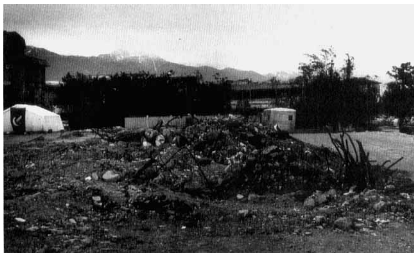
Fig. 1. The aftermath of the 13 March 1992 Erzincan earthquake.
