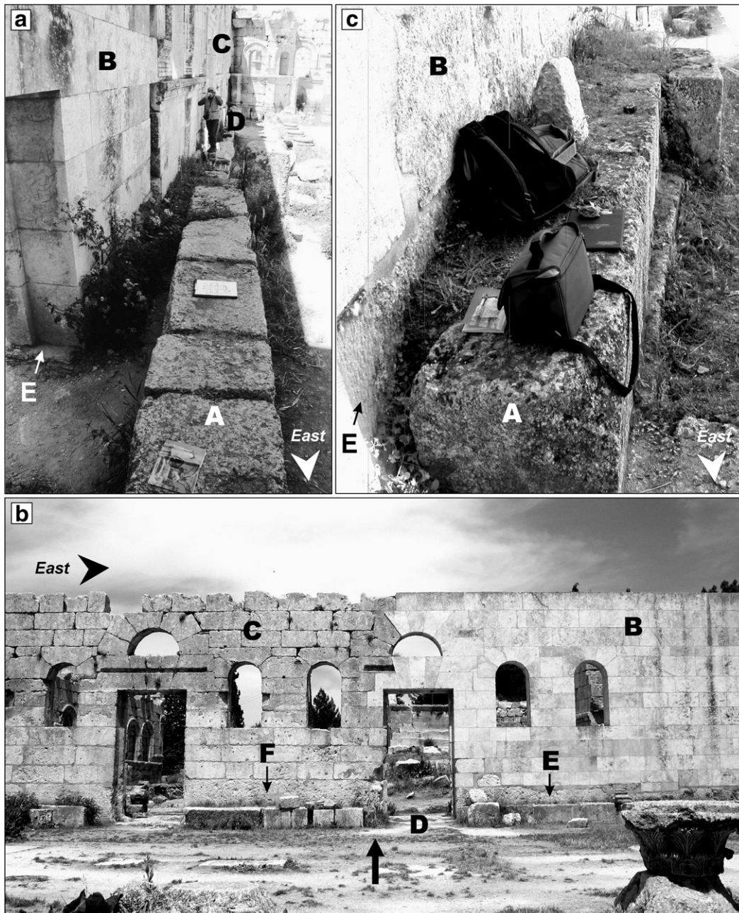
Fig. 18. Old wall fragments in the eastern wing of the main church a—the northern wall of the eastern wing, a view from the Prothesis. (A—the old wall, B—the wall with the masonry restored in the 20th century, C—the wall existing today with the old masonry, D—a part of the old wall fragment joining the wall existing today, E—old foundation, based on which the walls were reconstructed in the 20th century). b—the northern wall of the eastern wing: a view from inside (C—the wall existing today with the old masonry, D—a part of the old wall fragment joining the wall existing today, E—old foundation, based on which the walls were reconstructed in the 20th century, F—a part of the monolithic foundation hollowed in the bedrock) c—the southern wall of the eastern wing, a view from inside (A—the old wall, B—wall with the masonry restored in the 20th century, C—the wall existing today with the old masonry, E—based on which the walls were reconstructed in the 20th century).
